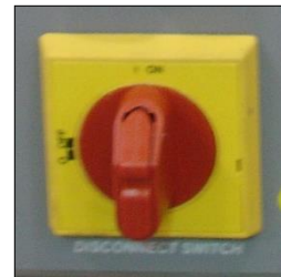
Figure 1. Disconnect Switch.
